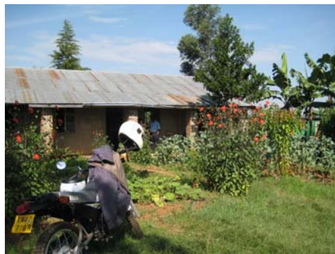
Madegwa Special Unit
